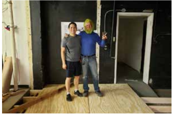
Gus & John install New Floor
